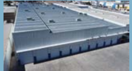
VTCW - P2, second plant built in 2022
