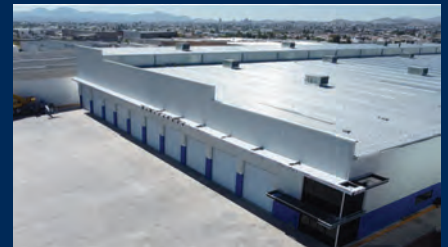
VTCW - P2, second plant built in 2022
