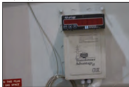
Electronic Temperature Monitor
