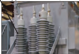
HV Bushings & Arrestors (Shipped demounted)
