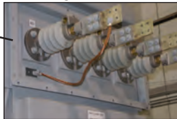
Side-Mounted LV Bushings
