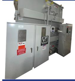
Base MVA – 6.705 Top MVA – 6.705 kV Rating – 34.5/34.5 Zig-Zag
